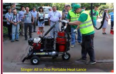
LAB Hot Air Lances blast out dirt & debris with Hot Compressed Air. They Draw out moisture from cracks without "over cooking"; lifting off oxidized surface leaving a warm, dry surface, properly prepared sealant adhesion.
